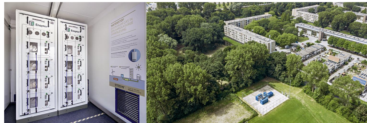
Residential heating with hydrogen - Rozenburg, The Netherlands
